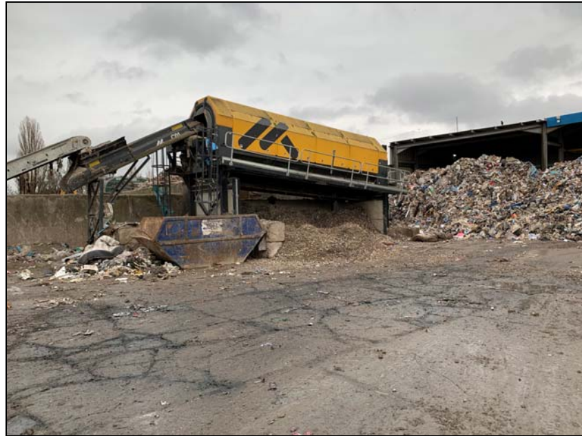
Plate 5: Picking station sorting bays for heavy inert waste
