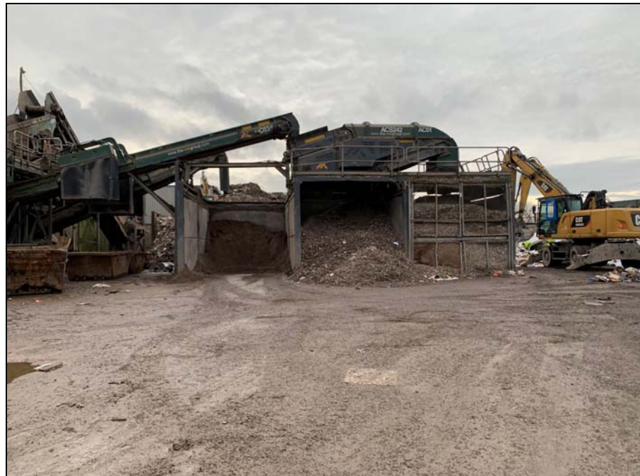
Plate 2: View of impermeable surface as required at the site
